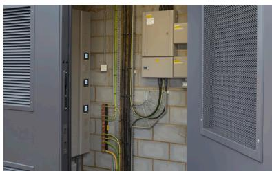
weather test ratings. These personnel and fire exit doors are fabricated from the best quality zinc-impregnated steel, offering extra protection from corrosion.
